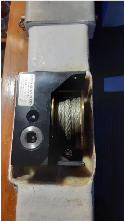
The New Winch in Position but Too High
