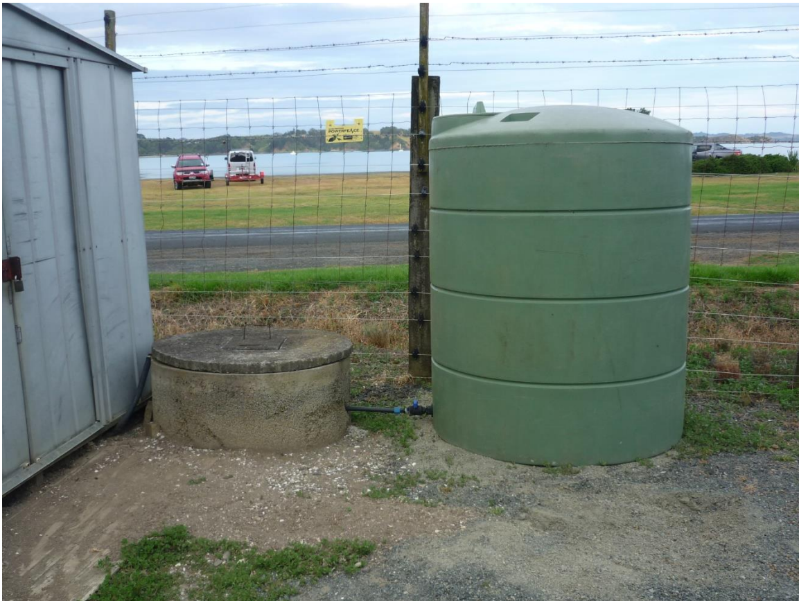
Concrete Well on the Left with the New Tank on the Right
