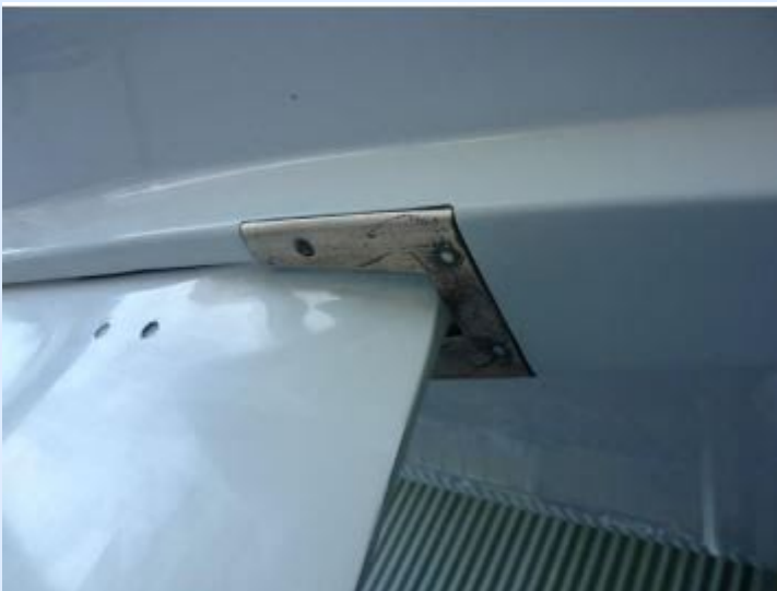
Aft end of the keel showing the keeper plate – all rejuvenated and back together
